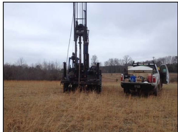
Photo 2. View from B-204 looking west
