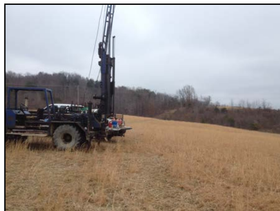
Photo 4. View from B-109 looking west
