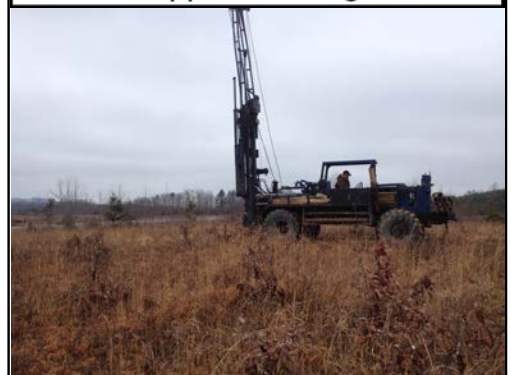
Photo of Approx. Boring Location
